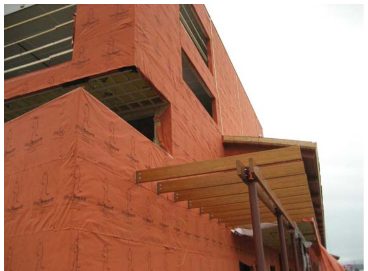
Designed for extreme weather installation, WrapShield SA Self-Adhered made an ideal choice for Waterfront Station located in the wintry Yukon Territory.
