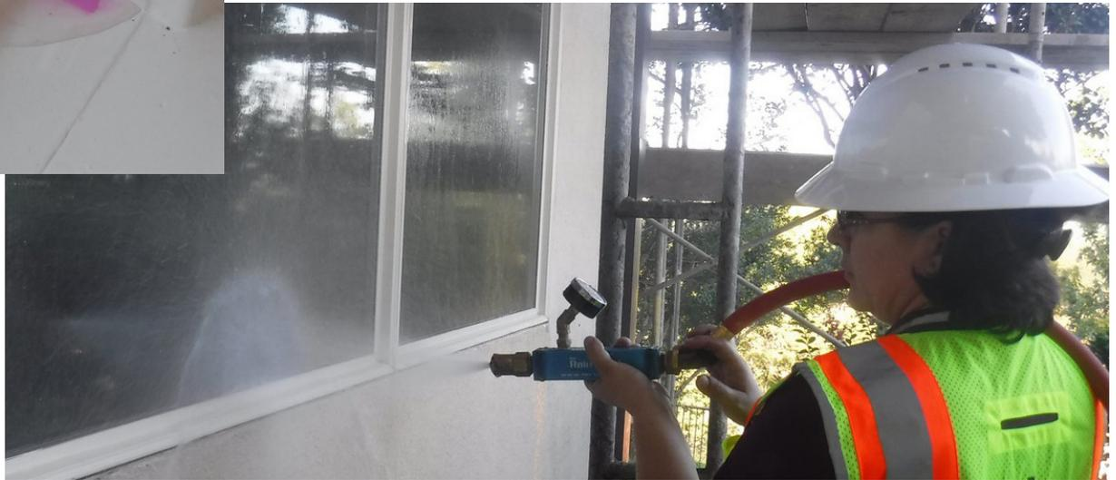
Using the Two-Part Simplified flashing system from VaproShield, the window penetrations were expertly installed to ensure long term moisture resistance.
