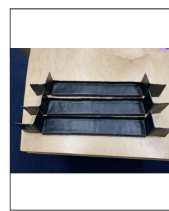
Sill Pan Flashing
