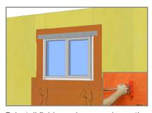
7. Install field membrane underneath 6" flap of sill flashing to create shingle effect, remove release film, adhere to
