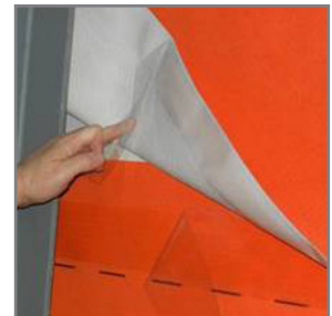
8. Begin joining horizontal seams by removing both release films (the underside of the overlapping upper course and the top side of the lower course).
