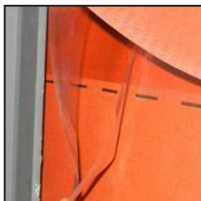
9. Line up both release films together so they can be pulled down the wall with one hand.
