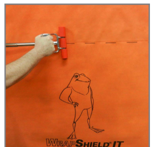
11. Immediately roll the integrated tape horizontal seams with floor roller to ensure full contact.
