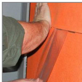
10. Use the opposite hand to smooth the two layers together as the release film is removed.
