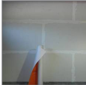
1. Begin installation at the base of the wall, progressing in a shingle fashion upwards.
