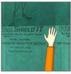
10. Optional for extreme exposure locations: Smooth out wrinkles with hand pressure and seal the adhesive strips using a hand roller.
