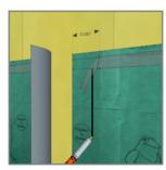
5. Remove release film from top of adhesive strip where flap overlaps.
