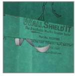
7. Optional for extreme exposure locations: Join horizontal seams by peeling back both release films, starting from where horizontal joint meets vertical joint.
