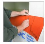
4. Slit material at corners to allow it to fold into the opening.
