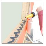
6. Using a sausage gun or DRY joint knife, apply VaproLiqui-Flash in a zigzag pattern on outer 2.75" of inside of rough opening.
