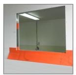
5. Fold flap into opening and adhere to inside surface, being sure to keep the lower 6" of release paper intact.
