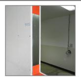
1. Cut and install WrapFlashing SA patches over pre-punched holes in metal studs, if present.
