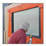
10. Apply VaproLiqui-Flash in a zigzag pattern on the wall face surrounding the rough opening.
