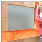
3. Install left & right jamb flashing with minimal stapling, allowing for later shingling with wall membrane.
