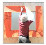
4. Install head flashing after left & right jamb pieces.
