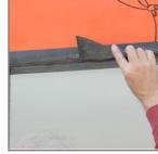
11. Immediately spread the VaproLiqui-Flash with a putty knife creating a 1" border around the rough opening (approximately 12 to 15 wet mils), paying special attention to the corners and edges.
