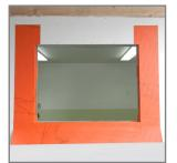
8. Install head flashing only after both left & right jamb pieces are fully adhered.
