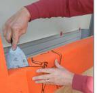
7. Immediately fold flaps into opening, pressing into the VaproLiqui-Flash with putty knife, spreading VaproLiqui-Flash evenly beneath WrapFlashing.
