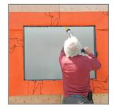
8. Using the sausage gun or DRY joint knife, apply a second layer of VaproLiqui-Flash over the folded flaps in a zigzag pattern on the inner surface of the rough opening.
