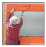
9. Immediately spread the applied material with a putty knife, fully embedding the inner flaps of WrapFlashing sill, right & left jamb, and head pieces, fully covering all inner surfaces of rough opening.
