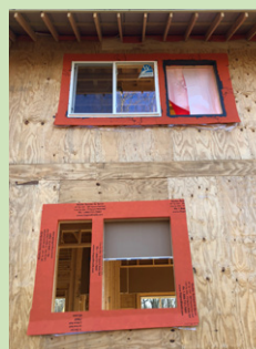
Window flashing in progress
