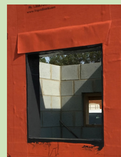
Rough opening ready for window installation, no reverse laps
