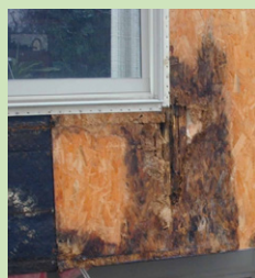
Rough Opening Leaks
