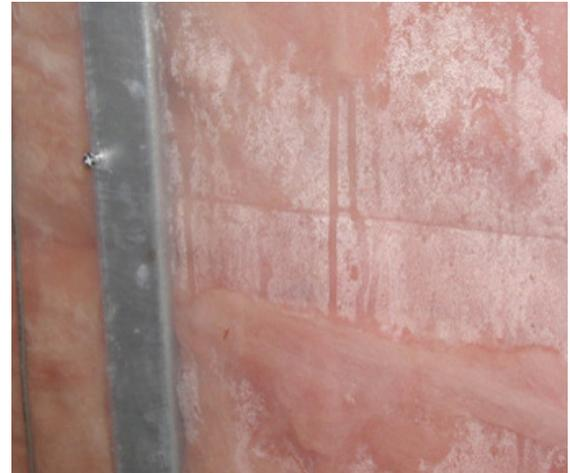
In the 1990's, air-conditioned homes with unventilated or poorly ventilated brick veneer were showing signs of condensation on the interior vapor barriers during the summer months. In the investigations that followed it was clear that the summer time condensation was in part due to reverse vapor drive.
