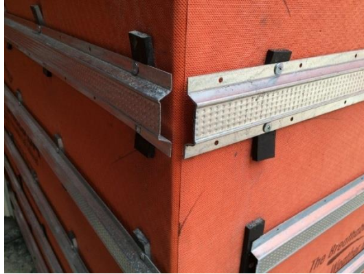
VaproShim™ (black), creates a small, effective 1/4" rain screen cavity, allowing for unimpeded vertical drainage of moisture away from the building envelope.
