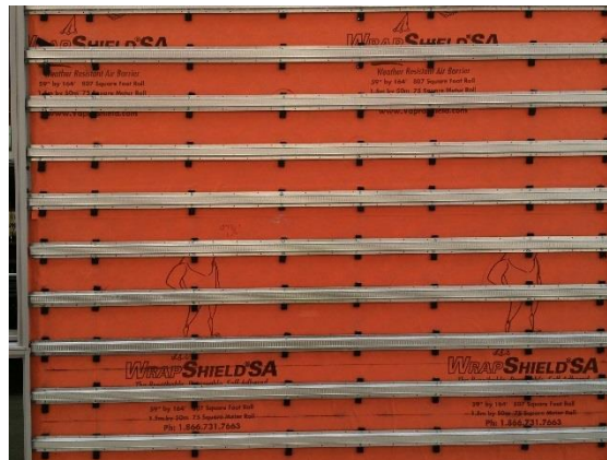
VaproShims used under horizontal cladding, seals fastener penetrations. The simple design adds minimal cost and helps to maximize building envelope drying capacity, for the life of the building.
