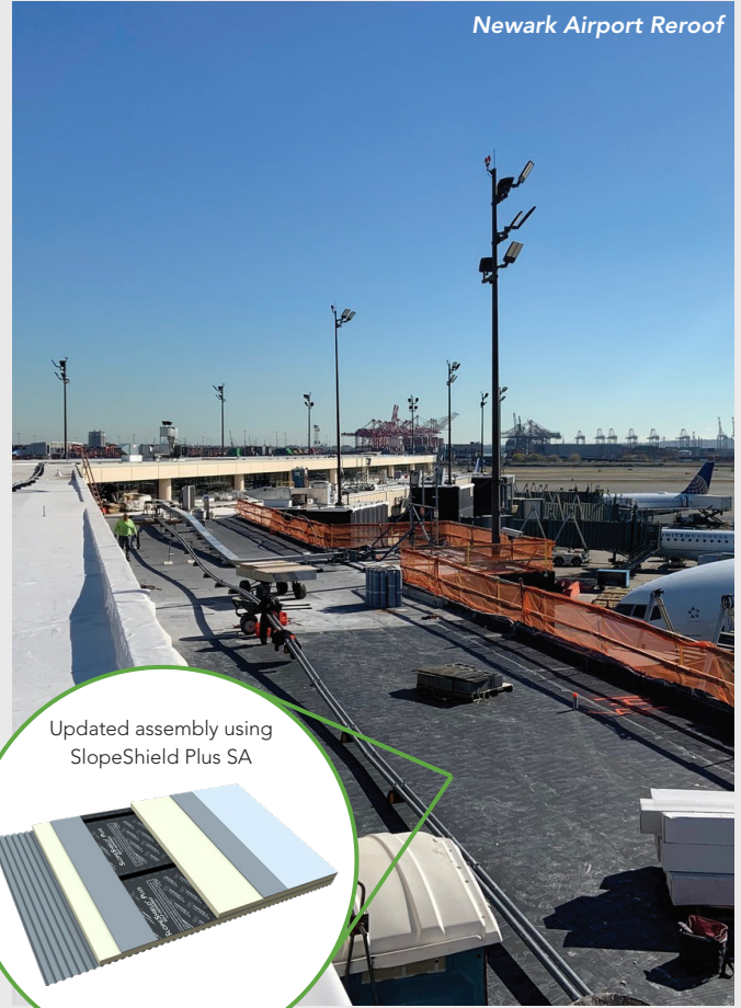
Install SlopeShield Plus SA allowing damp substrates to dry.
