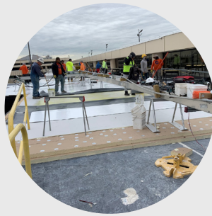
Install new insulation layer and roof covering.
