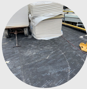
Install SlopeShield Plus SA allowing damp substrates to dry.
