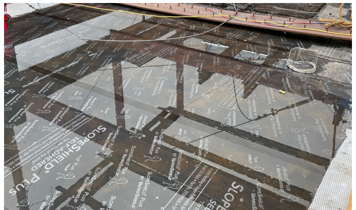
SlopeShield Plus SA even handles ponding water which can be easily swept away. Installation: Commercial Building, Seattle, WA
