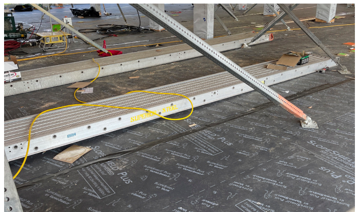
By protecting the interior floors with SlopeShield Plus SA, work can commence on the lower floors helping to keep the project on schedule. Installation: Multi-Family, Seattle, WA
