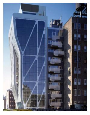
"The building's reverse-tapering form is more 'carved' or 'shaped' than set back," Denari explains. "But the inverted geometry was not just a dare on our part. It was an upfront response to the tough conditions of our site and its proximity to the industrial structure of the railway."
