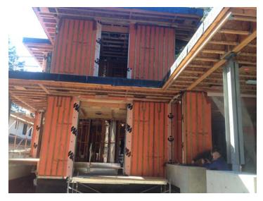
Over 10,000 sq. ft. (929 M²) of VaproShield products were installed on this private residence located in Vancouver, British Columbia. These products include: WrapShield Water Resistive Vapor Permeable Air Barrier Sheet, WrapShield SA Self-Adhered Water Resistive Air Barrier Sheet, RevealShield Black, UV Stable Water Resistive Vapor Permeable Air Barrier Membrane and VaproLiqui-Flash Vapor Permeable Liquid Applied Flashing.
