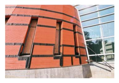
VaproFlashing Black was used for the open joint cladding.
