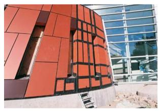
Left side of image shows cladding installed, right side WrapShield SA with VaproFlashing Black for the 1" open joints.
