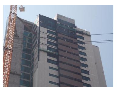
RevealShield IT Integrated Tape applied directly to the large cement tower, helping to dry out the cementitious substrate.
