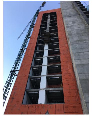
Approximately 30,000 sq. ft. of WrapShield SA Self-Adhered Water Resistive Vapor Permeable Air Barrier Sheet Membrane was installed in the construction of Alpino Condo Tower.
