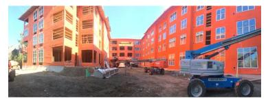
The Burnham & Ash Apartments is protecting their multi-million dollar investment with WrapShield IT (orange) Water Resistive Vapor Permeable Air Barrier Membrane.
