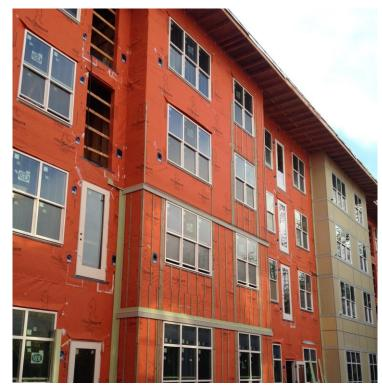
A mechanically attached, water resistive, vapor permeable air barrier membrane, WrapShield IT features integrated tape at the horizontal seams and easily creates the shingled effect for optimum air and water tight horizontal joinery.
