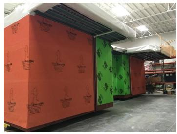
WrapShield SA Self-Adhered WRB/Air Barrier (orange) was installed on 20 modules at the American Modular Systems factory in Manteca, CA.
