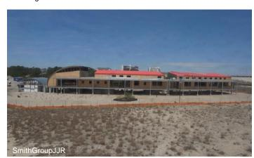
Slopeshield SA Self-Adhered (red) was installed under the 50year zinc shingles.
