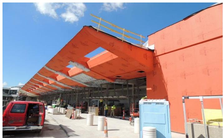
*WrapShield SA easily adheres to multiple substrates effortlessly accommodating complex installation conditions.*
