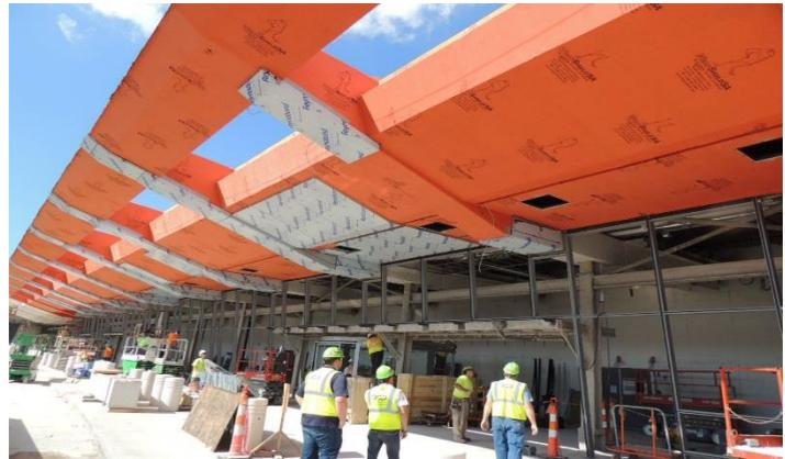
*Free of harmful VOC's and entirely self-adhering, VaproShield's WrapShield SA Self-Adhered was easily installed on the detailed, overhead soffit structures. Conventional products would have dripped down onto installation crews.*
