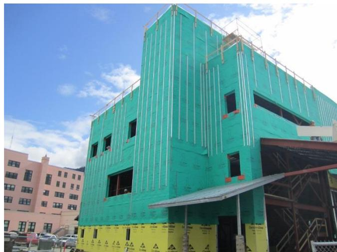
Over 10,000 sq.ft. of WallShield Water-Resistive Barrier Sheet was installed.
