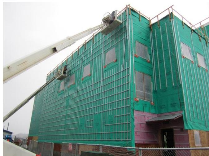
Rain Screen Design and 3D Flashing Elements were used during the installation of WallShield.
