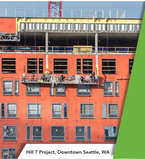
Time and Labor Saving Application All weather installation, no special joint treatment, primers or installation equipment ever required.
