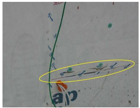
In the above photo note the dark line of debris at the horizontal seam which continues to the vertical seam.
