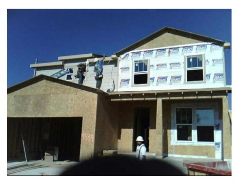
If the seams are going to be taped this generally occurs after the entire house is wrapped or after several courses of wrap are installed. Since most areas of house wrap are over wood-based sheathing, leaks at the seams may go undiscovered for years.
