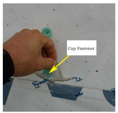
In the photo above you can see the debris carried by the water that has penetrated the "seal" created by the seam seal tape due to the cap fastener preventing the tape from making a complete seal. You can see that the water has run horizontally along the seam taking the path of least resistance.
