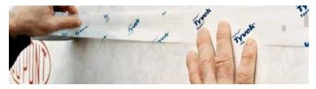
The horizontal seam tape is installed lapping over both layers of wrap. This means that the seam tape installation creates a reverse lap at the top of the tape. While this reverse lap might not result in leakage in laboratory conditions, in the field the installation of the tape is not always done properly. At times the wrap is not clean when the tape is
