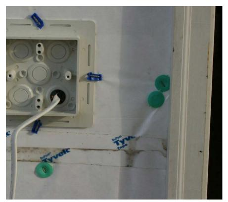
In the photo above the debris from the water intrusion can be seen at the wrinkle in the wrap. Note that the wrap is wrapped into the door frame so water can migrate horizontally past the door frame and into the interior.
