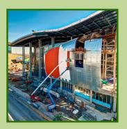
Over 400,000 Sq.Ft. of WrapShield SA Self-Adhered Water-Resistive Vapor Permeable Air Barrier sheet membrane was used on the construction of the new \$415 million Music City Center in Nashville, TN. Total land area is 16 acres and total square footage of this project is 2.1 million Sq.Ft.
