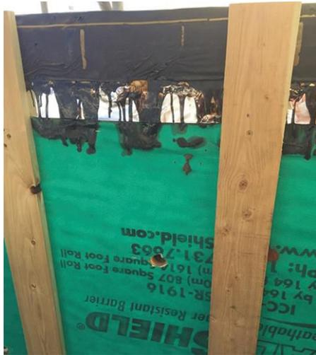
Figure 3: An example of wall to roof transition with material compatibility issues.
