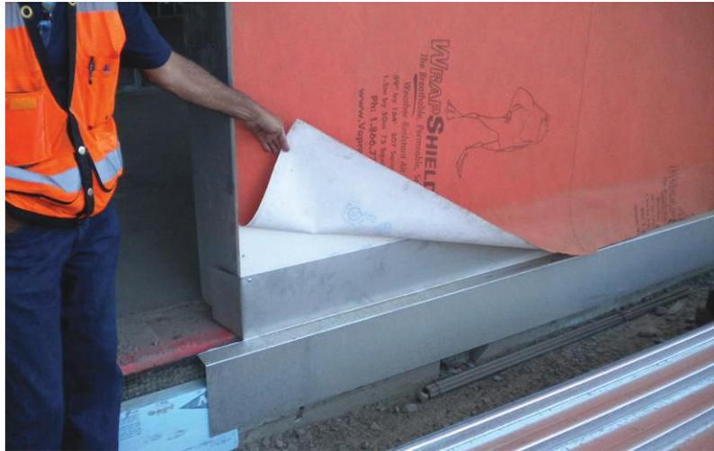
Figure 4: An example of an improperly detailed through wall flashing observed during a site observation walk.
