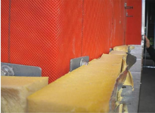
Figure 5: An example of a wall installation with an improperly designed rain screen. Note the rigid insulation installed directly over the face of the WRB/AB preventing proper drainage.
