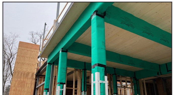
4. Connect and/or install wrapped post/column to wrapped beam. Use VaproTape as required on seams.
