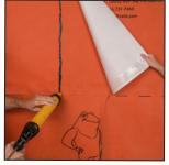
5. Apply VaproBond Adhesive Sealant in a single bead down the membrane to the bottom of the sheet.
