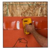
2. Install with SS staples in the top 2" above the Integrated Tape. Avoid stapling in the tape area.
