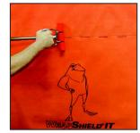
12. Immediately roll the integrated tape horizontal seams with floor roller to ensure full contact.
