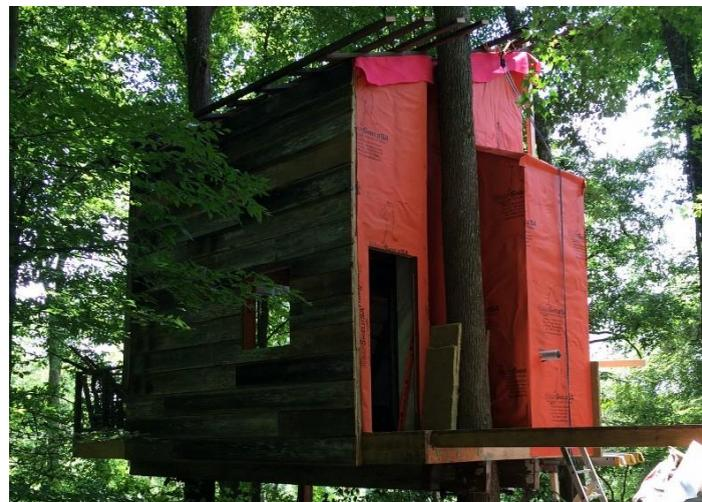
*Two hundred year reclaimed barn wood clads the treehouses. By using rain screen design and VaproShield membranes the treehouse building envelope is well protected from moisture intrusion.*
