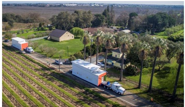
WrapShield SA Self-Adhered's durability and ability to be exposed for up to six months, contributed to the complex shipping process from Manteca to Lodi, CA.
