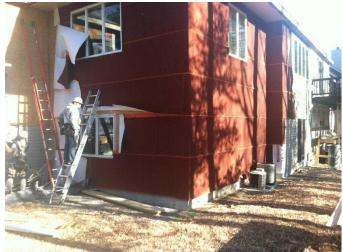
Over 150,000 sq.ft. of WrapShield HS Water Resistive Vapor Permeable Air Barrier Sheet with Drainage Matrix was installed during the renovation of the Wayland Condos.
