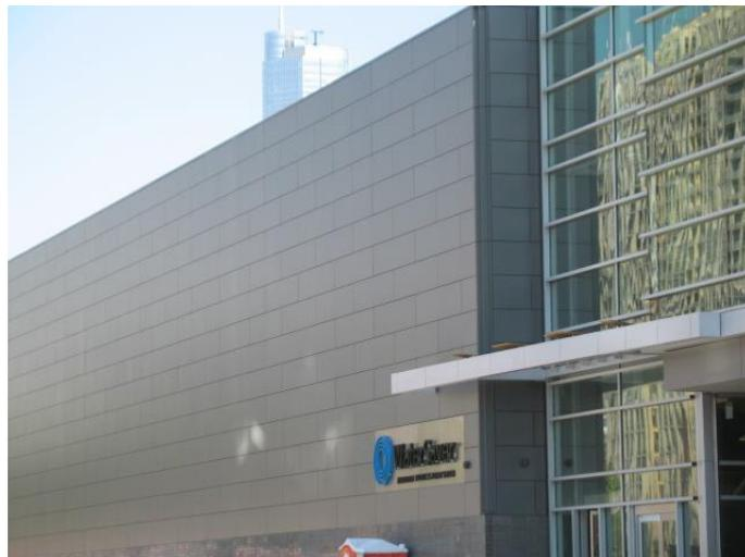
VaproFlashing was used behind the open joints on the reclad.
