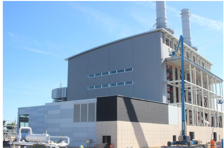
Over 10,000 sq.ft. of RevealShield SA Self-Adhered (black) was installed on the Holland Energy Park.
