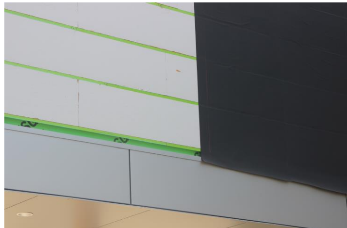
RevealShield SA Self-Adhered was installed over USG gypsum sheathing.
