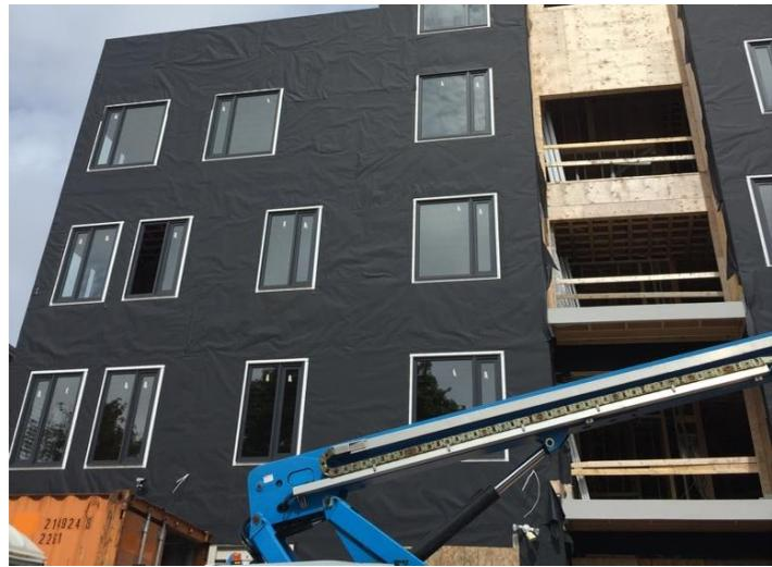
*Approximately 35,000 sq. ft. of RevealShield UV Stable Water Resistive Vapor Permeable Air Barrier Membrane was installed on the new Harris East Condos.*
