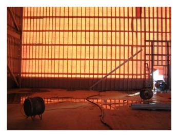
Even with moisture building up inside due to propane fueled heat, the WrapShield surface stayed completely dry.
