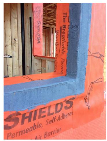
VaproFlashing and VaproLiqui-Flash were used on all window and door openings reducing installation time and ensuring breathable but air-tight seals.
