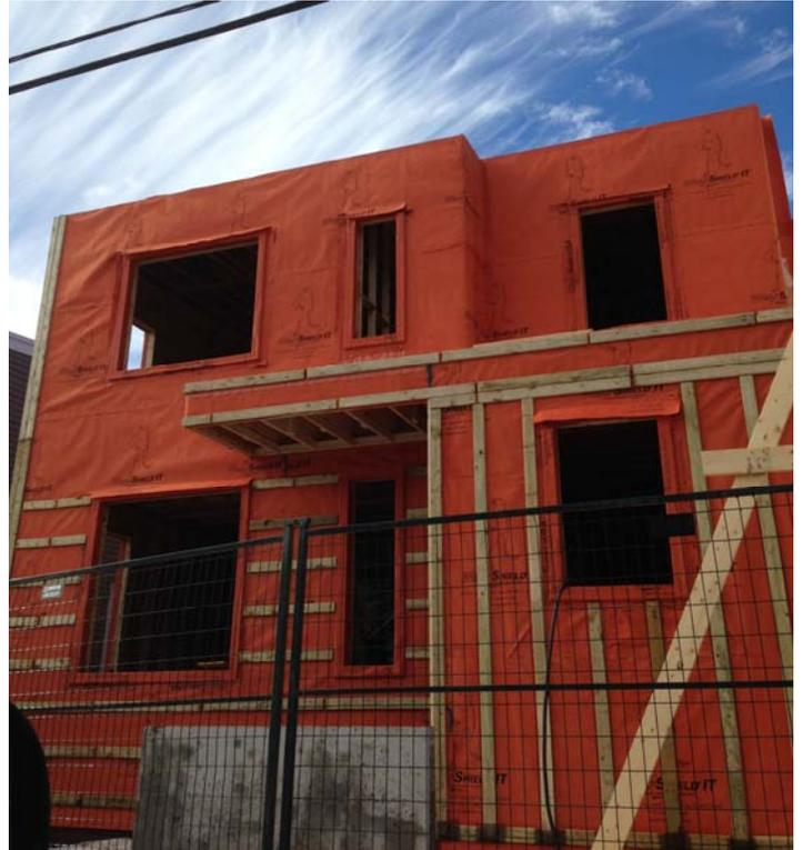
Over 3,000 sq. ft. (278.71 M<sup>2</sup>) of WrapShield Water Resistive Vapor Permeable Air Barrier Membrane was installed on this modern urban home located in Halifax, Nova Scotia.
