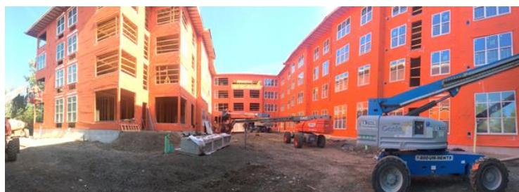
*The Burnham & Ash Apartments is protecting their multi-million dollar investment with WrapShield IT (orange) Water Resistive Vapor Permeable Air Barrier Membrane.*
