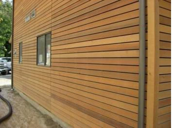
Detail of open joint rain screen design Prodema cladding with VaproFlashing Black
