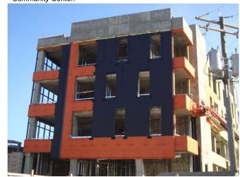
A single layer of RevealShield (Black), UV Stable Weather Resistive Vapor Permeable Air Barrier Membrane was installed behind open joint Trespa Panels.
