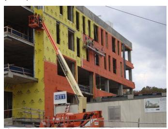
Over 56,000 sq. ft. of WrapShield Water Resistive Vapor Permeable Air Barrier Membrane Orange was installed.
