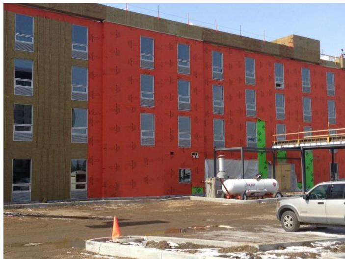
Over 2,787 m<sup>2</sup> of WrapShield SA Self-Adhered Air Barrier (orange) was installed on the new "hip and humble" Home2 Suites.
