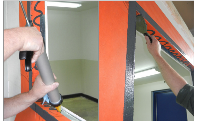
Quick and easy to apply around rough openings, VaproLiqui-Flash bonds without primers, is waterproof and breathable. Tapes, frequent cutting and precise corner installation have been eliminated saving valuable field labor time.
