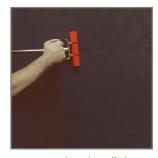
11. Immediately roll the integrated tape horizontal seams with floor roller to ensure full contact.
