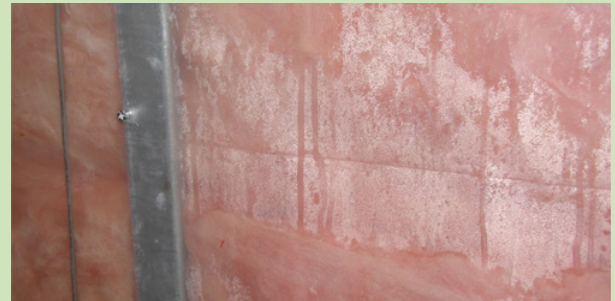
Image shows poorly ventilated wall with condensation.
