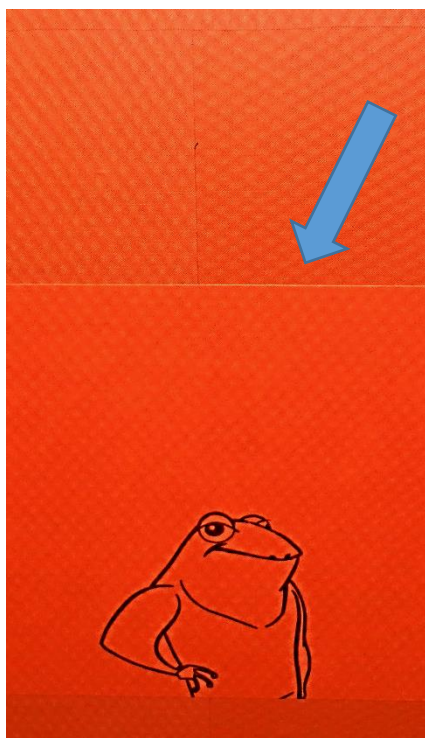
Figure 2 , Reverse lapping noted by arrow.
