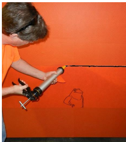
Figure 3 , VaproBond™ sealant added to the reverse lap edge.
