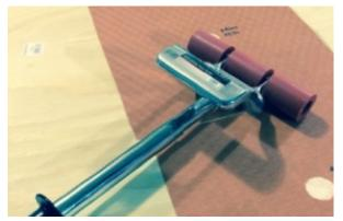
**Figure 1**, Ensure the reversed lapped **WrapShield SA Self-Adhered** is bonded to the surface by utilizing a hand roller such as the Superior-Hand-Roller-80-R32-M.
