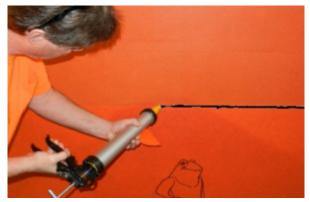
Figure 3, apply a bead of VaproBond™ sealant the full length of the seam
