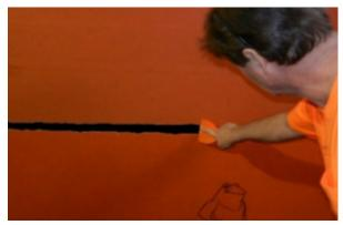
Figure 4, Feather the bead of VaproBond™ using a hand trowel
