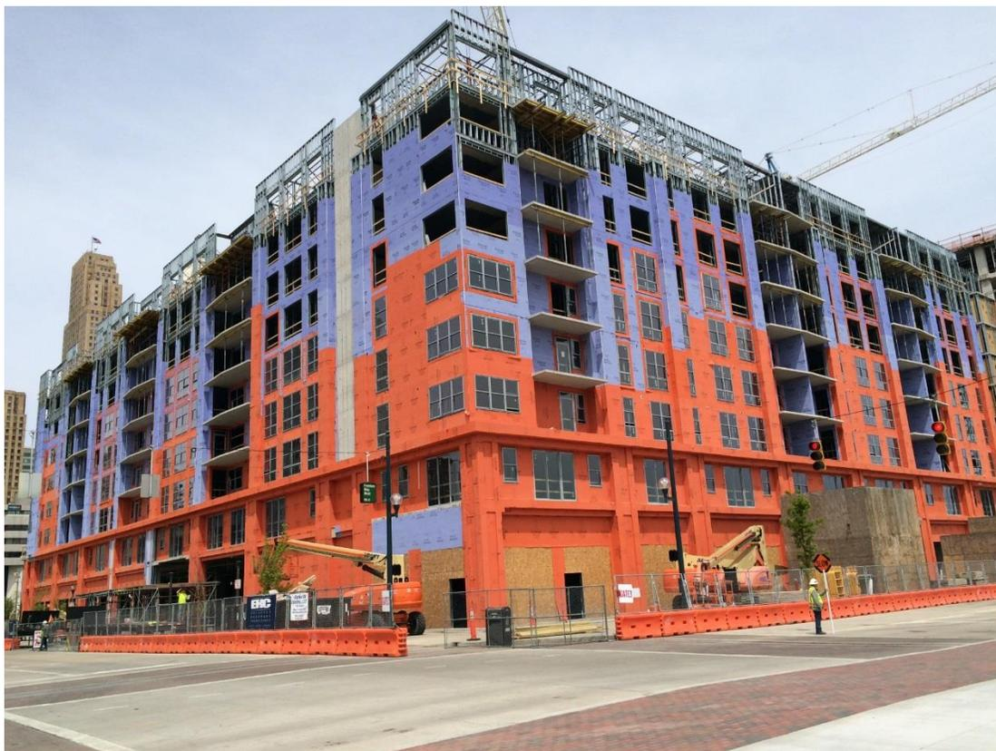
*WrapShield SA Self-Adhered is applicable for all climates and weather conditions, and can be installed in temperatures as low as 20°F (-6° C) which made VaproShield a better choice than the fluid-applied product that would have been impractical and expensive to be applied in the windy, cold conditions of this project.*
