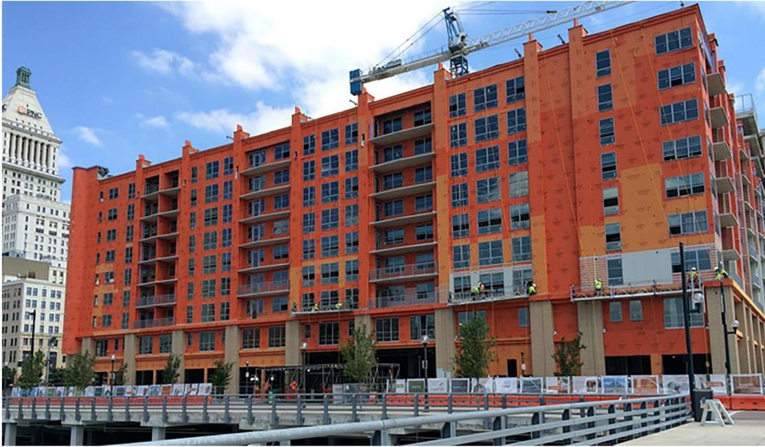
*150,000 sq. ft. of WrapShield SA Self-Adhered Water Resistive Vapor Permeable Air Barrier sheet membrane was installed on The Banks Phase II Mixed-Use Building after initially choosing a fluid-applied product.*
