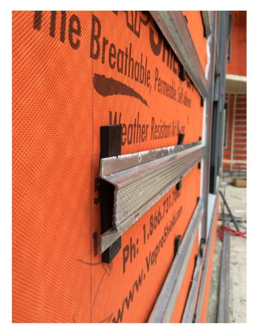
VaproShims used under horizontal cladding attachment created a small, effective ¼" rain screen cavity, allowing for unimpeded vertical drainage of moisture away from the building envelope.
