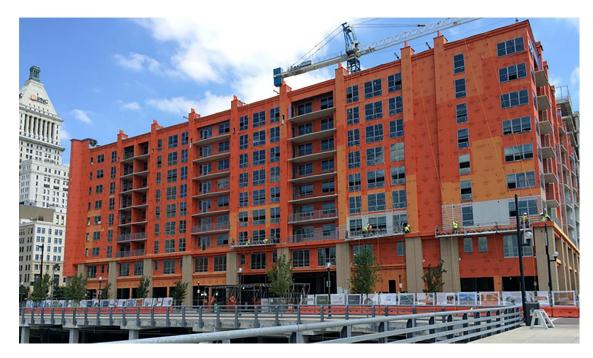
150,000 sq. ft. of WrapShield SA Self-Adhered Water Resistive Vapor Permeable Air Barrier sheet membrane was installed on The Banks Phase II Mixed-Use Building after initially choosing a fluid-applied product.
