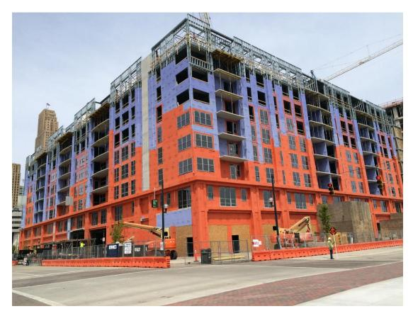
WrapShield SA Self-Adhered is applicable for all climates and weather conditions, and can be installed in temperatures as low as 20°F (-6° C) which made VaproShield a better choice than the fluid-applied product that would have been impractical and expensive to be applied in the windy, cold conditions of this project.
