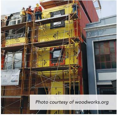
RevealShield was installed as part of an open joint rain screen system with Parklex cladding. Windows were flashed with WrapShield which was also installed behind James Hardie<sup>®</sup> Commercial Board Siding Products.
