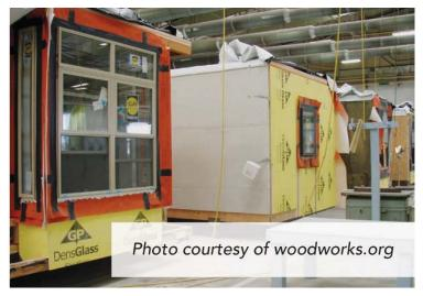
Using prefab modular construction, installation of the modules took one week and the entire project was completed in six months – from ground breaking to completion.
