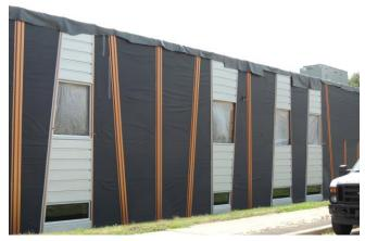
Approximately 10,000 sq. ft. of (black) RevealShield IT Integrated Tape; UV Stable, Water Resistive Vapor Permeable Air Barrier Membrane, was installed on the IBEW Local 58 Detroit Zero Net Energy Demonstration Center
